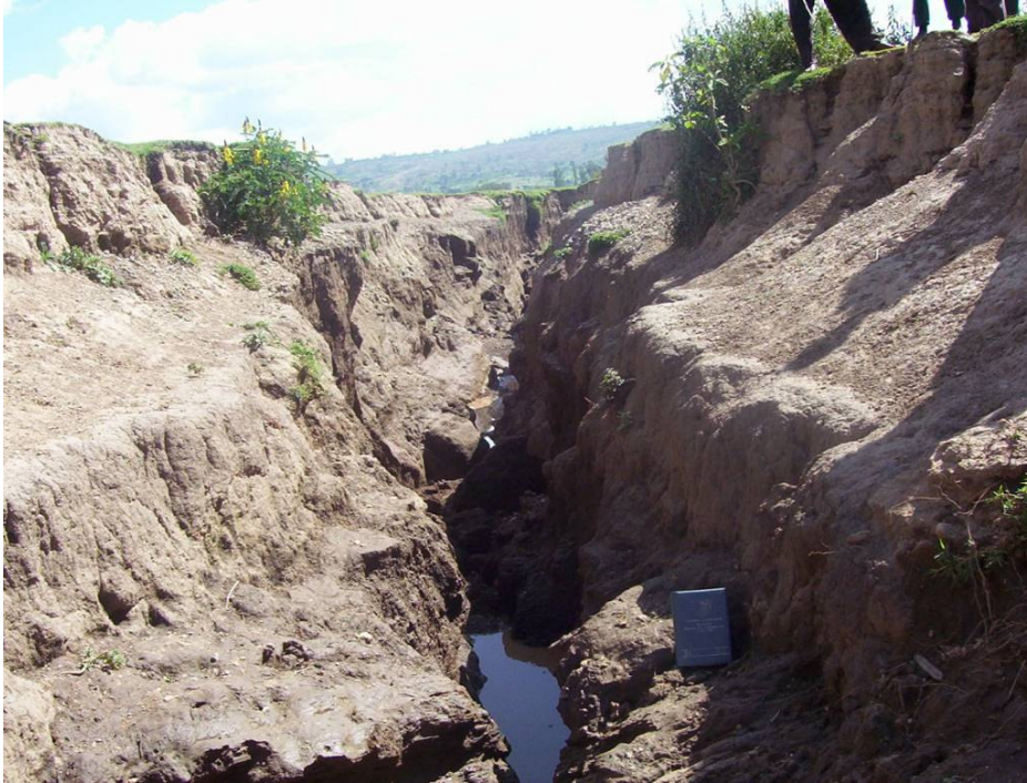
Figure 16 Some of the recent ground cracks (1996-1998) on lake Awassa catchment (Muleti area)
