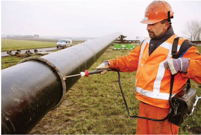
Figure 55 Sample of inspection activity
