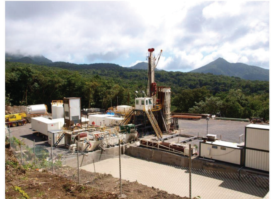
Figure 45 Rotary rig drilling slim holes up to 1500m (Source: ISOR)
