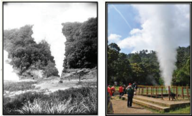
Figure 9 KMJ-3 Well Drilled by the Dutch 1926 (source: courtesy of PGE)
