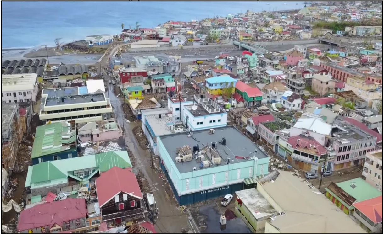
Image 01: Part of the area affected by flooding that was not mapped on the inventory. Sediment deposition can be seen along the streets with damaged buildings.
