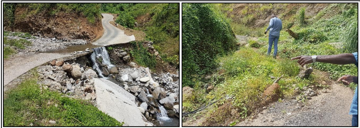
Figure 5.4: Road conditions in the area of Petite Savanne. The area has difficult accessibility and public connection infrastructures are in poor quality.
