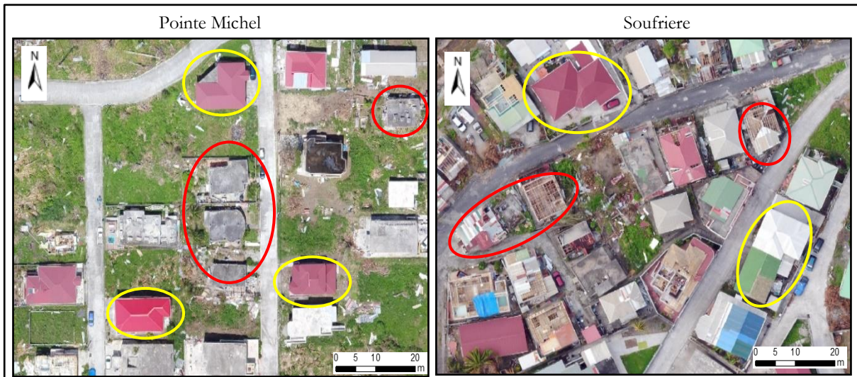
Figure 3.4: Damage pattern to buildings in two locations of Dominica. The figures depict a comparison of the situation between damaged houses and houses with little to no damage. Red circles indicate buildings with construction design that suffered more damage. Yellow circles depict buildings with little to no damage and possible better construction design.
