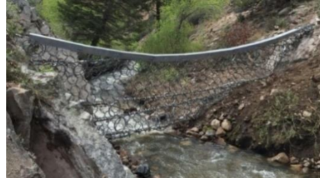
Figure 6-8 Example of retention structures. Retention net of high resistance for the capture of solid load. Source: Wendeler (2016)
