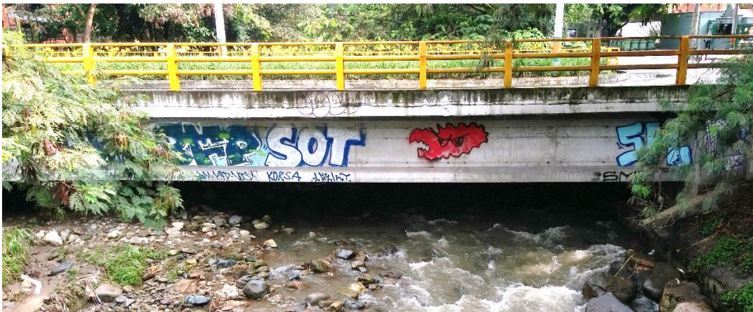
Figure 3-1. Obstruction caused by the presence of a concrete slab under bridges inside the channel of the Ayura stream.
