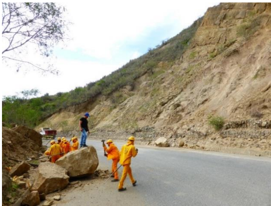
Figure 2.4: Maintenance staff working on manually disintegrating a boulder from the upper slope beside the road in Pasto; Photo source: CJ van Westen (2018)
