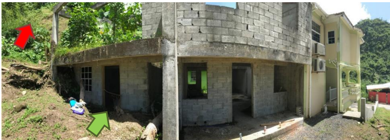
Figure 3.10: Debris source indicated by the red arrow; green arrow points to the flooded room in Figure 3.11
