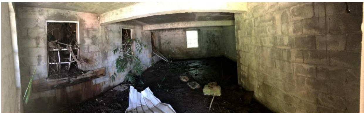
Figure 3.11: Flooded room with debris in the windows resulting in an even layer of soil in the room
