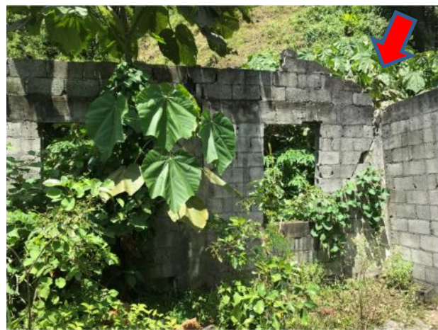
Figure 3.12 & 3.13: (Top) The second-floor of the affected wall on Building 2 was buckling at the red arrow from the accumulated debris; (Bottom) the affected wall and frame was cracked, at the red arrow, due to debris in Figure 3.12
