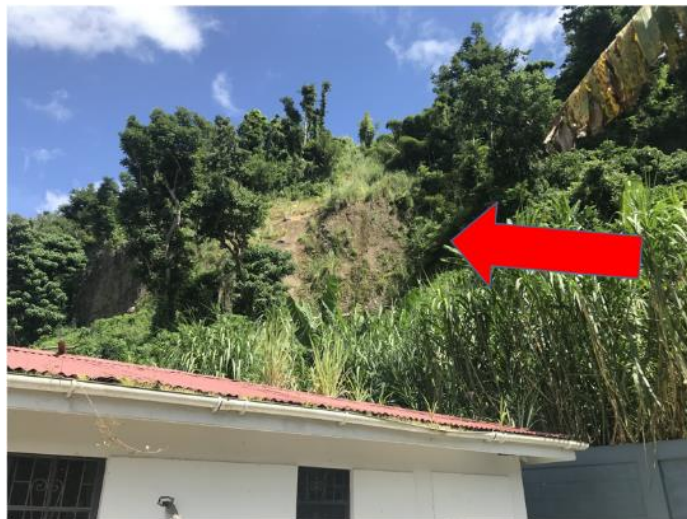
Figure: (Left) Debris slide erosion visible from the driveway (Right) Flooding stains along the walls
