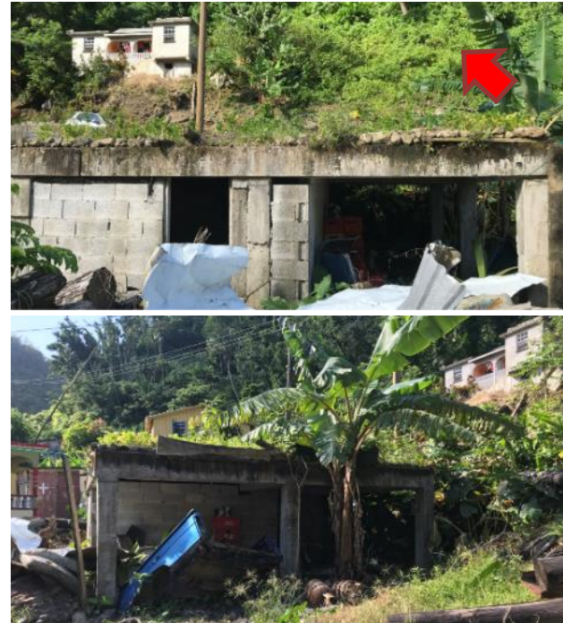
Figure 3.6 & 3.7: (Top) Building 1 is missing an additional timber framed second-story, and the debris slide mobilised from across the road identified by the red arrow; there is a car parked on the road below building on the hill. (Bottom) Side profile of Building 1; there are cracks visible where the walls do not touch the frame or ceiling slab, and debris accumulated around the buildings
