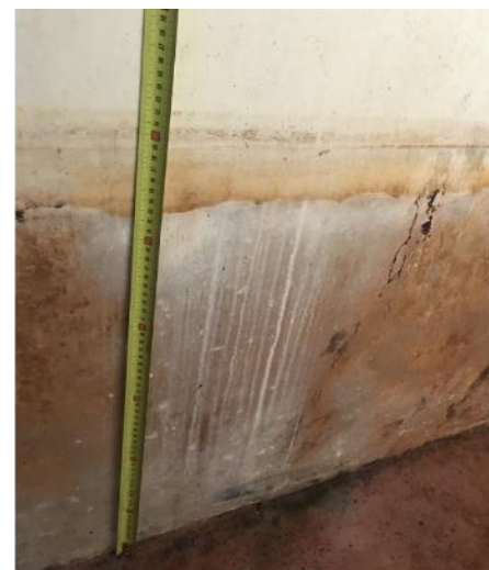
Figure: (Left) Debris slide erosion visible from the driveway (Right) Flooding stains along the walls
