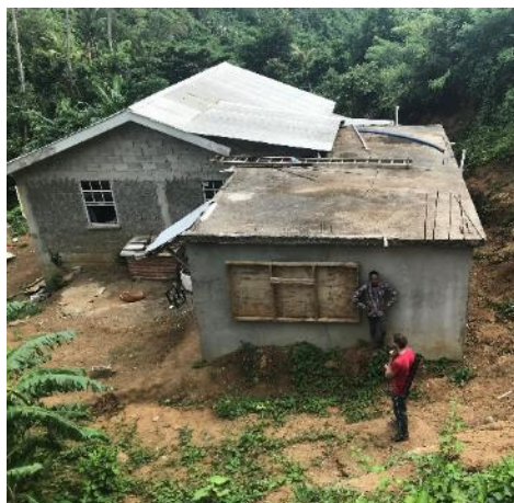
Figures 3.3 & 3.4: (Left) Single story concrete block building affected by a debris slide; (Right) single-story building, raised on a reinforced concrete frame, affected by debris flows and a sediment stream.
