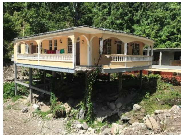
Figures 3.3 & 3.4: (Left) Single story concrete block building affected by a debris slide; (Right) single-story building, raised on a reinforced concrete frame, affected by debris flows and a sediment stream.
