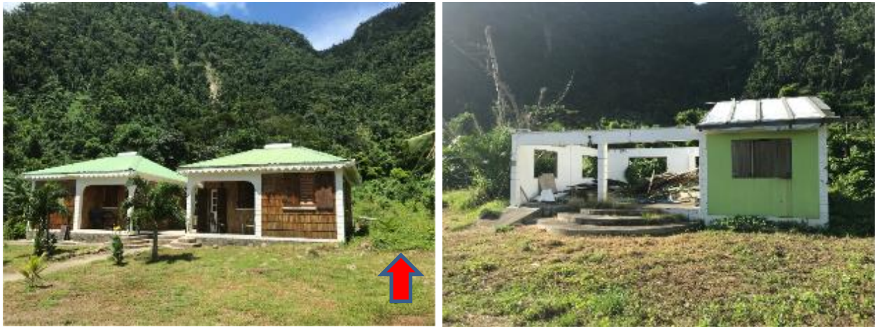
Figure 3.32 & 3.33: (Left) Assessment 8, at Site 21, has been excavated in the front but accumulated debris is left over on the right side; indicated by red arrow (Right) Assessment 9 is a storage facility, the boarded window is part of an inaccessible room
