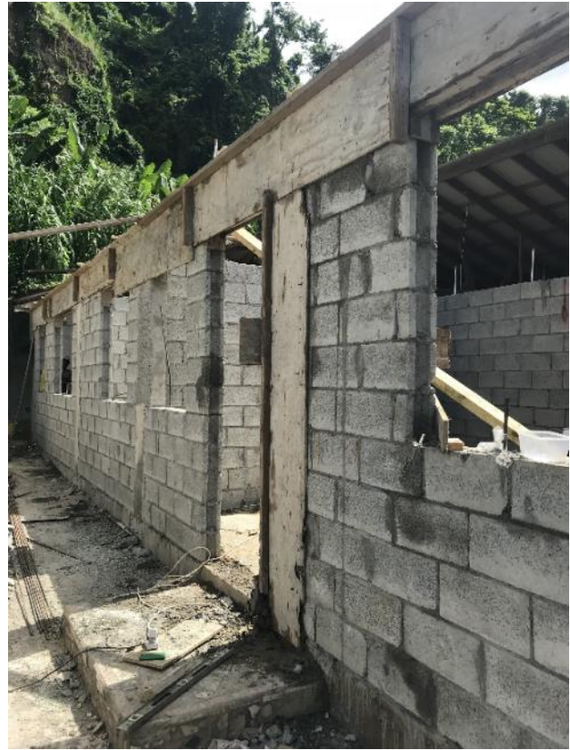
Figure: Building 10 being constructed to look the as it did before Hurricane Maria
