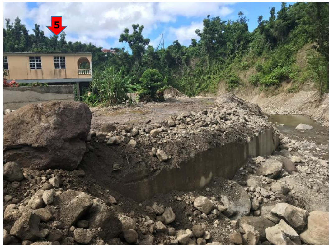
(Bot-Right) Two meter tall retaining walls along the river being excavated
