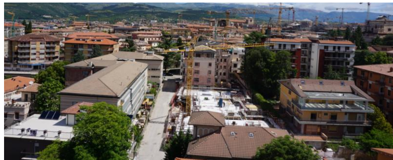
Figure 3-2 L'Aquila one of oblique images to show the area
