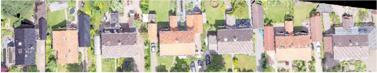
Figure 5-15 UAV Orthomosaic for Possible roofs, dormers and chimneys found by the segmentation search
