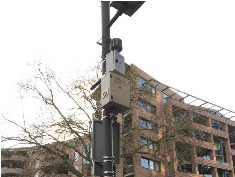
Figure 2. ILM airbox installed in the city of Eindhoven.
