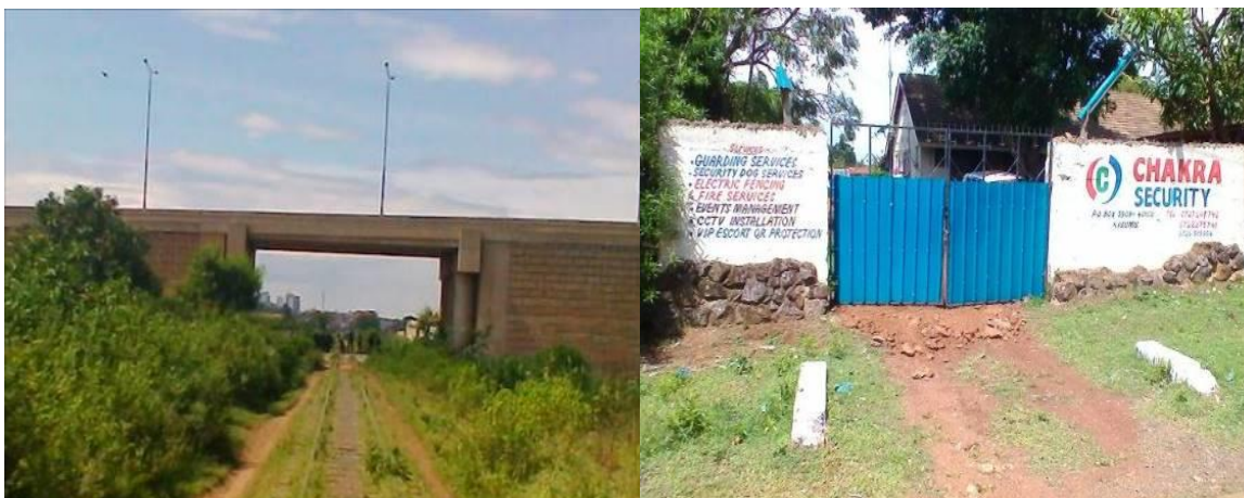
Figure 4-14: Overpass with railway line beneath (left) and Security firm in Tom Mboya (right)
