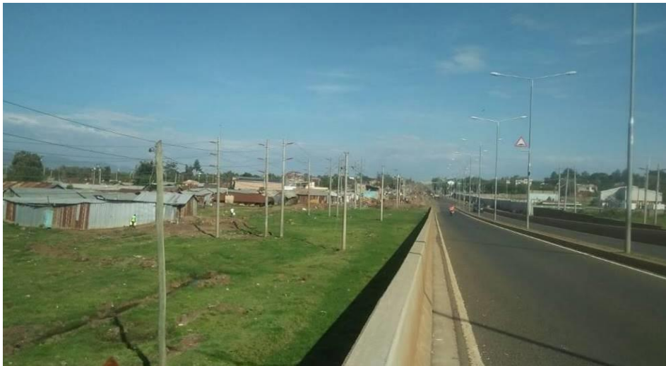
Figure 4-10: A section of the Bypass in the study area with street lights
