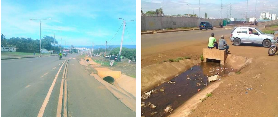
Figure 4-12: Improved drainage system along the bypass in the Study Area
