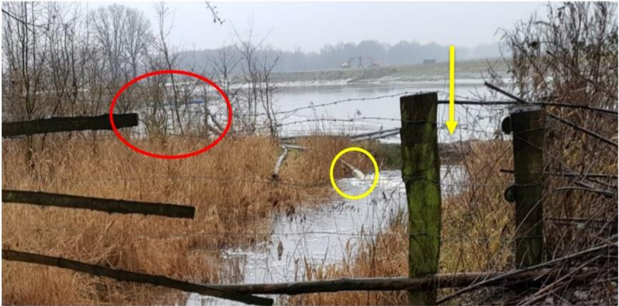
Figure 30: Water Management in progress at Aamsveen's Camping area
