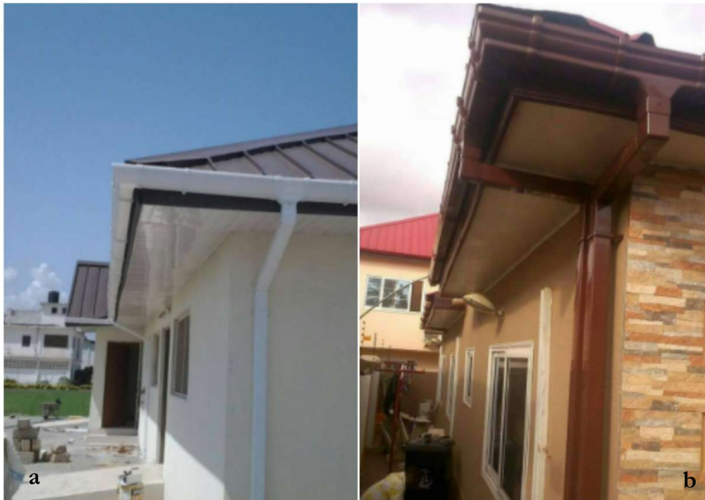
Figure 4-18: first example of "rain gutters" (a) and second example of "rain gutters" (b)
