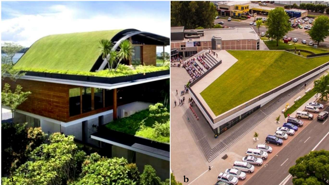
Figure 2-1: First example of a green roof (a), second example of a green roof (b) Source: (Fremantle Roofing Services, 2020; Architecture & Design, 2016)
