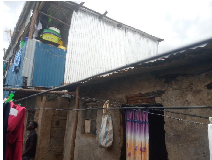
Figure 38: Image depicting three types of building material in one area. On the right is a stone-walled house with a second storey for an iron shack; on the left, a mud with concrete plastering house.
